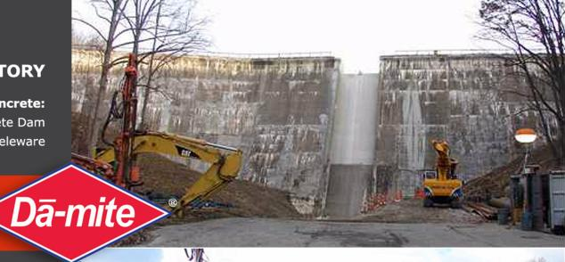
Da-mite was used to crack reinforced concrete to aid in demolition of a Dam. Drilled 2" holes with Sandvik 700 Track Drill, Depth: 11-12 feet per lift. Drill Pattern was 18" centers, due to the way rebar was laying in the concrete.
